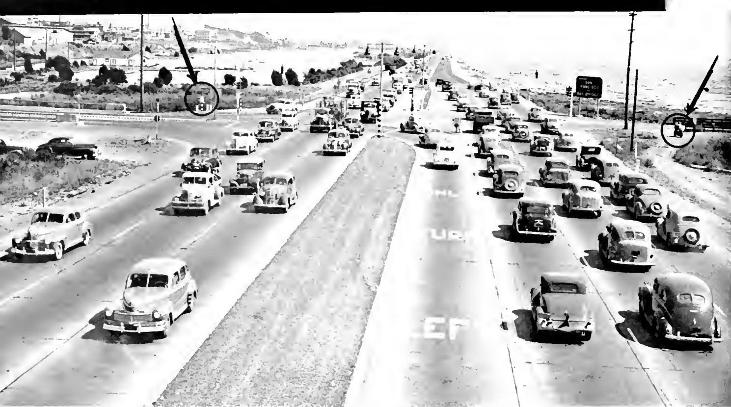
Scene at intersection on East Shore Highway, Contra Costa County, where an electric monitor (in circle at left) governs through and turning movements on six lanes of heavy traffic watched by officer on bike shown in circle at right
